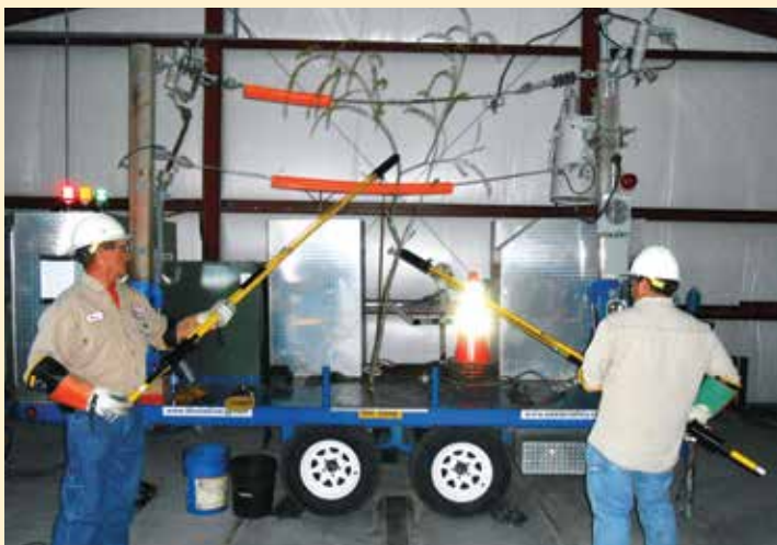
Linemen Bruce Loy (left) and Nathan Porter don special rubber gloves and use hot sticks to protect themselves from becoming part of the electric path to ground while removing a branch from a live power line during a safety demonstration.
