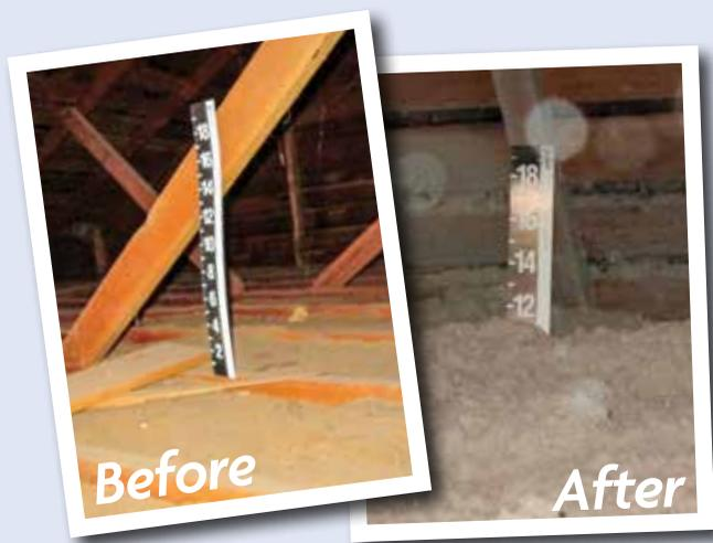
Varna's attic had less than an inch of insulation prior to the Energy Efficiency Makeover. Matt Hoisington, C&V Home Improvement, increased the insulation to the recommended 10-12 inches.
